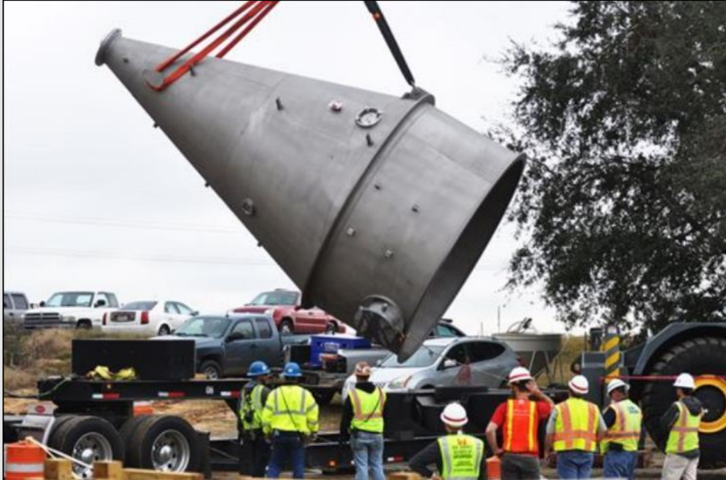
Figure 29. Speece cones delivered as part of the Savannah Harbor Expansion Project environmental mitigation (US Army Corps of Engineers 2017)
