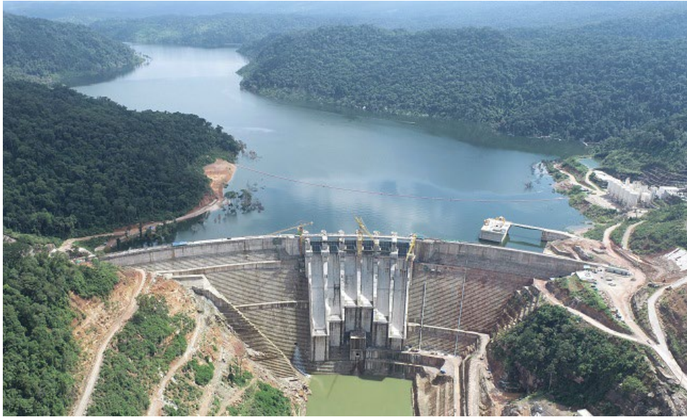
Figure 2: Nam Theun 1 RCC dam
