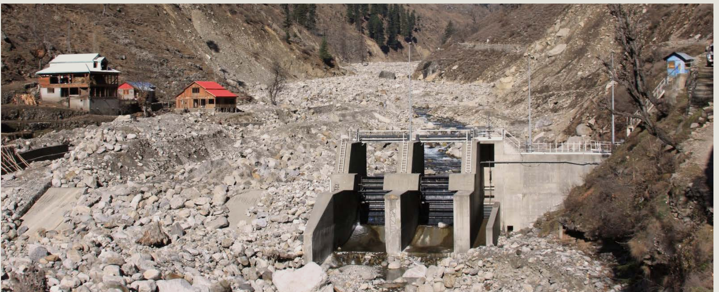
Weirs must be capable of safely passing floods without being damaged.
